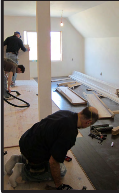
Members of Team #3 laying flooring at Hope Center in Yamamoto
