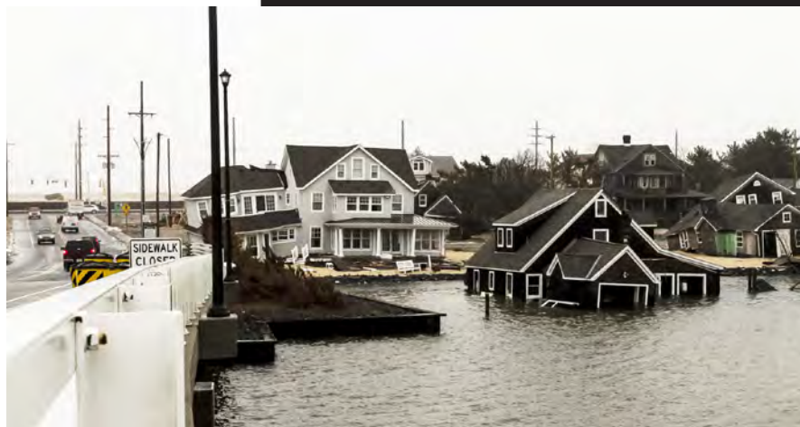
Devastation on the barrier island
