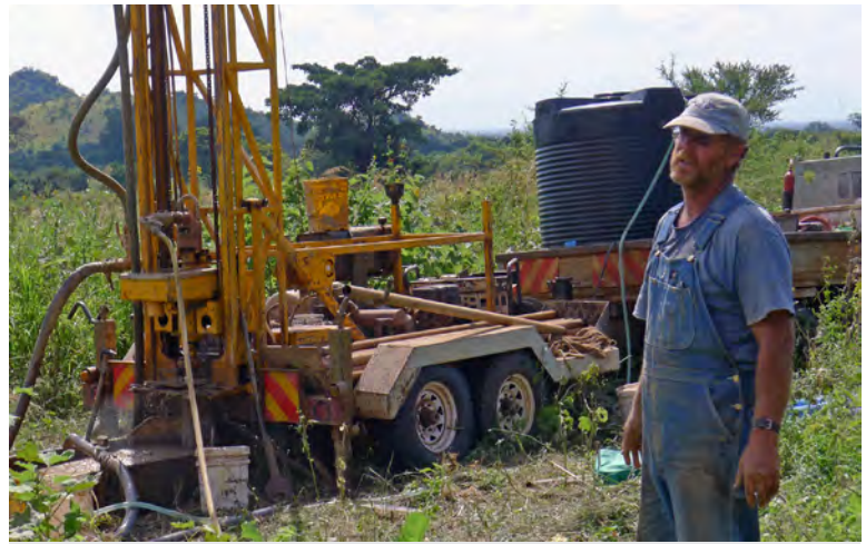
Bob Wright with his well-drilling rig
