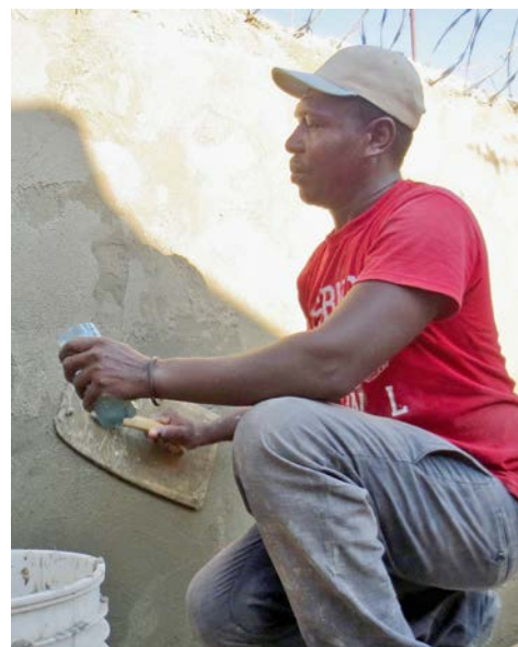
Elissaint plastering the La Gonâve guesthouse wall
