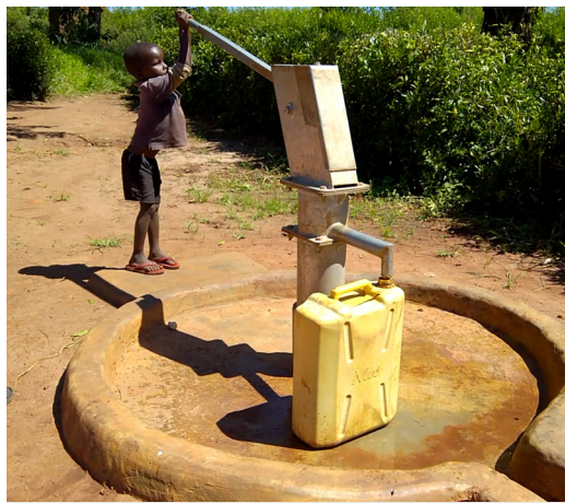
Pumping water from a borehole
