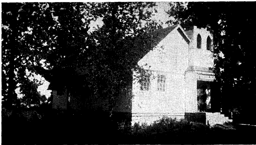
Building, as yet unfinished, of the Old Stockbridge Orthodox Presbyterian Church at Morgan Siding near Gresham, Wisconsin.
