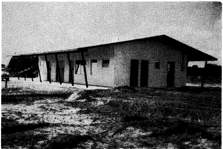
Hialeah Chapel: New building of the Orthodox Presbyterian Church in Hialeah, Florida, which was dedicated on January 27. The work is under the direction of the Rev. Robert Lucas. This structure, of southern type construction, is the first unit of a proposed plan that will include auditorium and educational buildings. The surrounding area is rapidly being built up with middle income homes.
