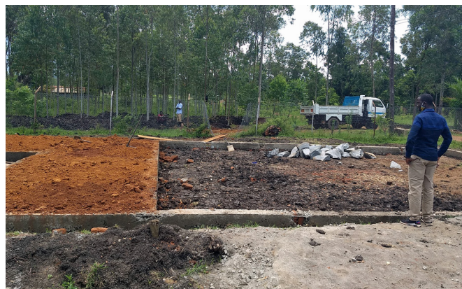
Pavilion construction underway
