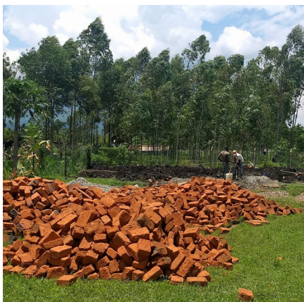
Bricks for KST's new pavilion
